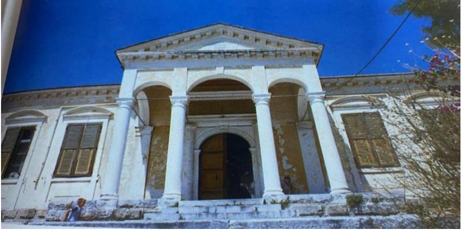
Picture 1.1. Suleymaniye Madrasah Entrance Gate (Çelikkol, 1992, Picture 294).
